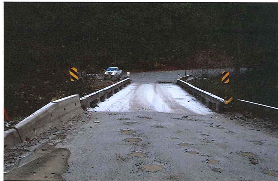
CK-2091 Approach Right Bank
