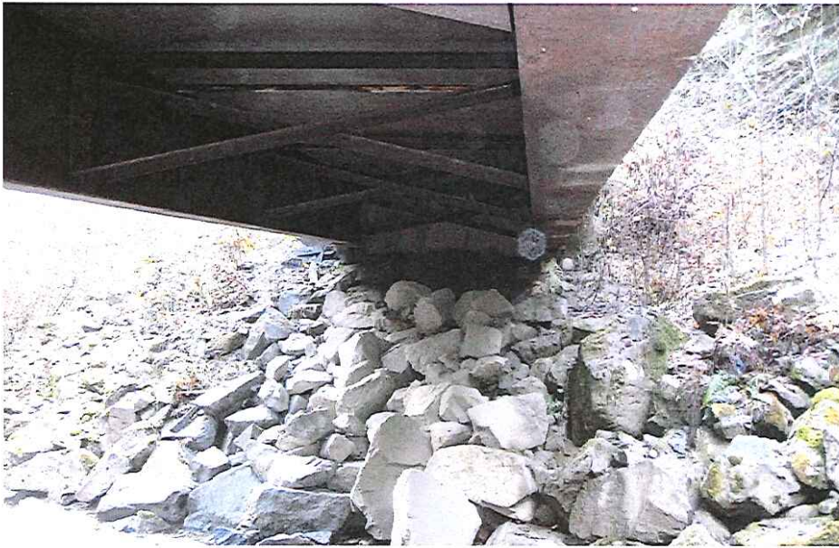
CK-2091 Abutment Right Bank
