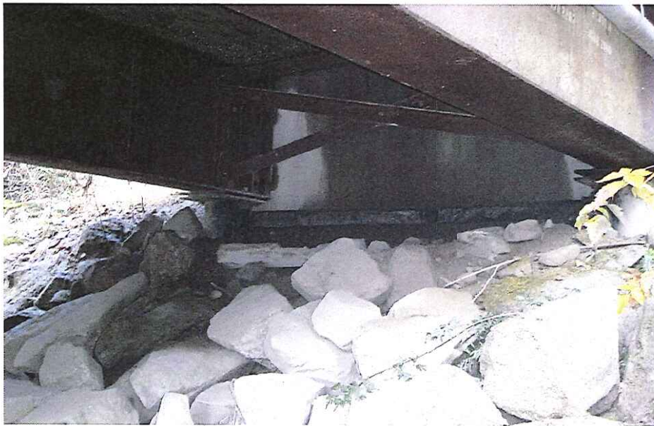
CK-2091 Abutment Left Bank
